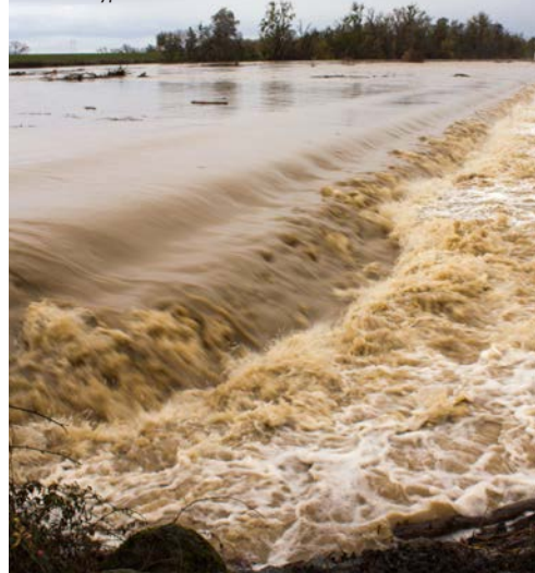
Tisdale Weir spills water from the Sacramento Weir into the Sutter Bypass
