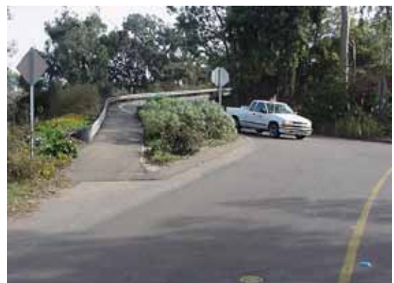
Curb extension and asphalt sidewalk, Del Mar
