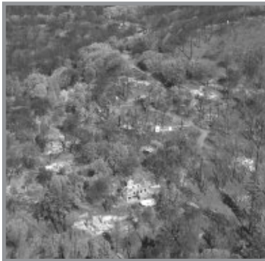
Aerial photo showing vegetation and structure loss following the 2003 Cedar Wildfire.
