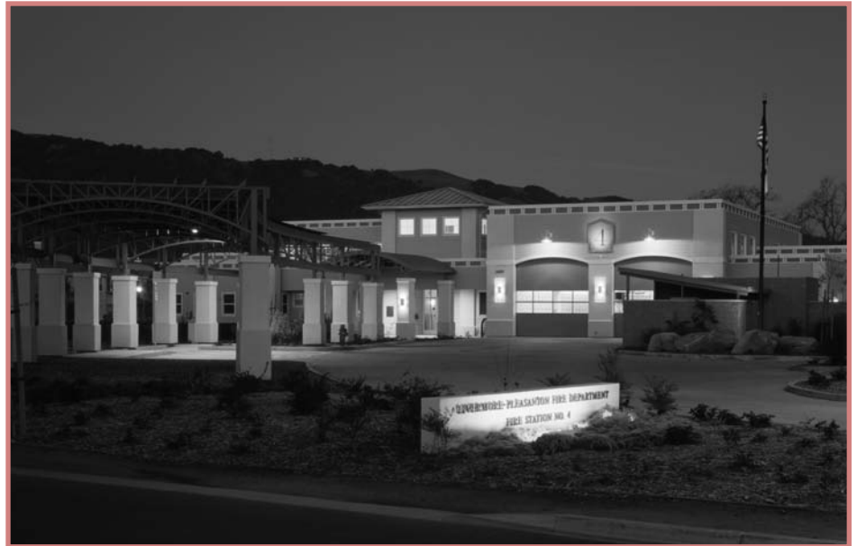
LEED Gold Fire Station, Pleasanton, CA
