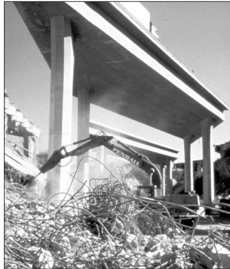
Constructed in the 1960s, the La Cienega-Venice Undercrossing of the I-10 (Santa Monica) freeway was one of seven bridges that collapsed. These non-ductile columns failed in shear and then collapsed under the weight of the bridge. (Photo: Jack Moehle)
