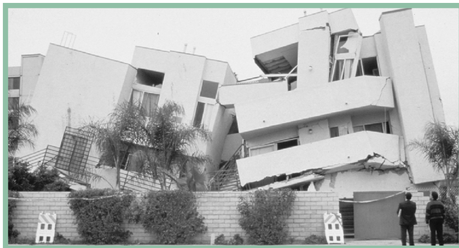
A woodframe residential building on Sherman Way collapsed inward over unbraced entrances to a garage. (Photo: Chris Arnold)
