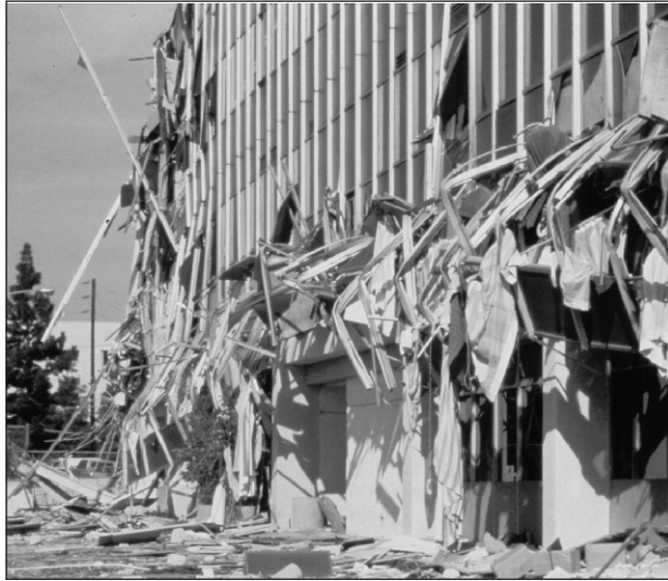
The Kaiser Permanente building in Granada Hills suffered a complete collapse of its second story. (Photo: Lloyd Cluff)
